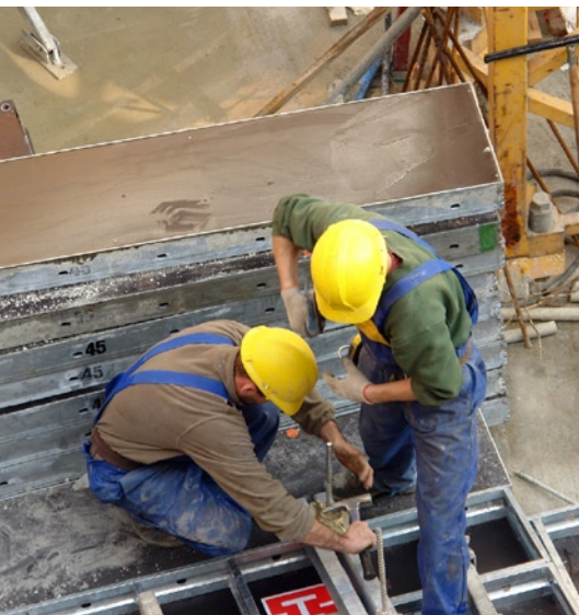
Monitoring – from 1 July 2007 DIAC and OWS will have increased powers to access premises and documents. Are you ready for an unannounced site visit?
